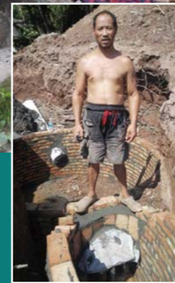
刘新武和在建的沼气池 Mr. Liu Xinwu and his biogas unit
